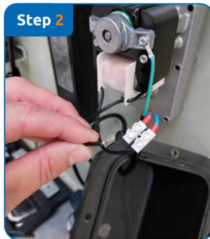
Unscrew the electric wires and remove them from the terminal block.
